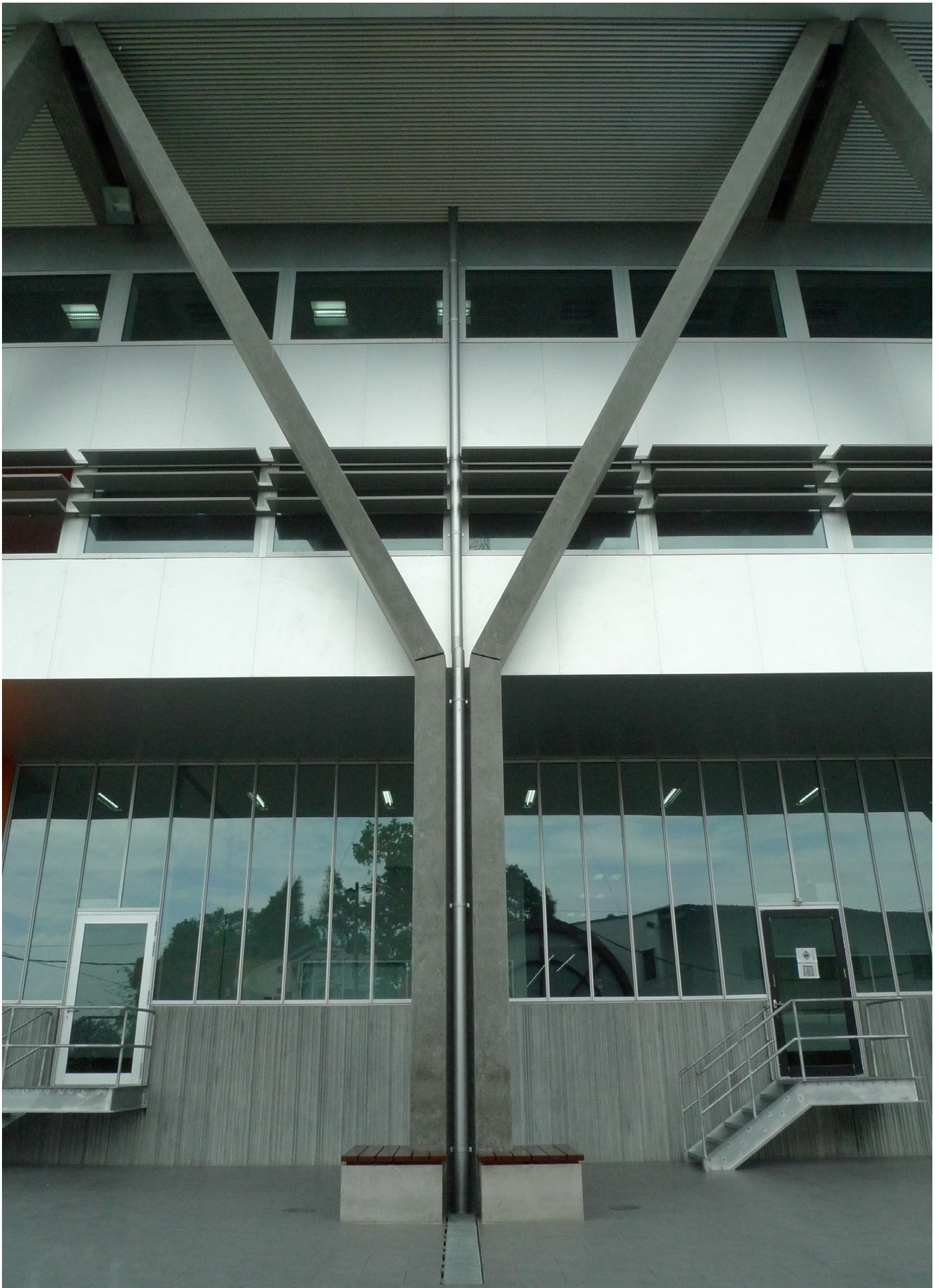
B.Braun Production Building - B3, Extension. Penang. Malaysia
