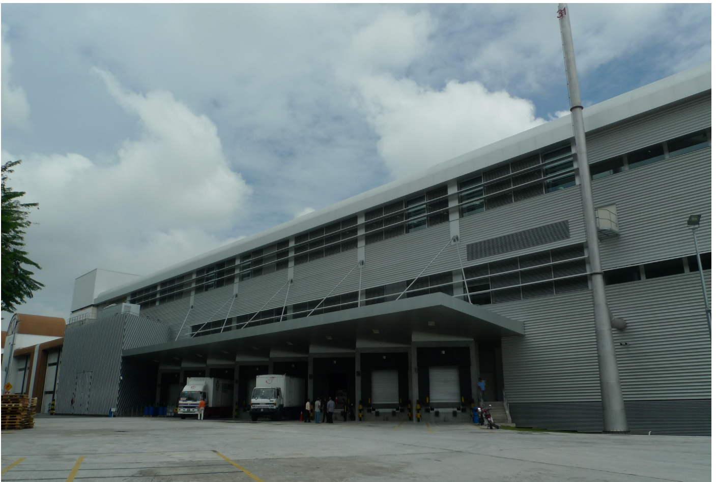
B.Braun Production Building - B3, Extension. Penang, Malaysia
