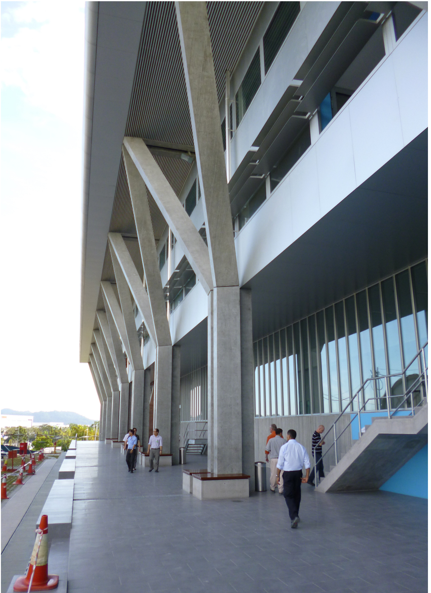
B.Braun Production Building - B3, Extension. Penang. Malaysia
